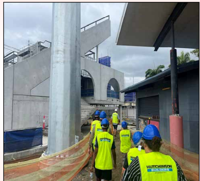
Site visit / Tour of the Browne Park construction
